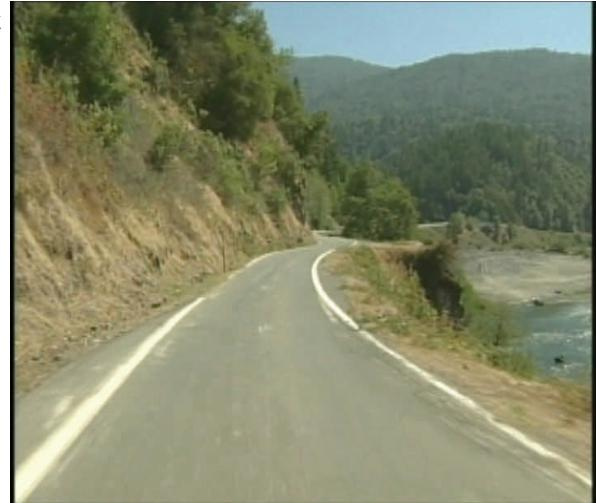
At times reservation roads are located on steep terrain with dangerous embankments. These hazardous conditions may result in fatal accidents during unruly weather conditions and/or when a driver is distracted. Some accidents can be prevented if the roads are equipped with guard rails, reflectors, and other safety devices that guide drivers through dangerous environments caused by bad weather and existing conditions that are already dangerous and made worse by weather conditions.
